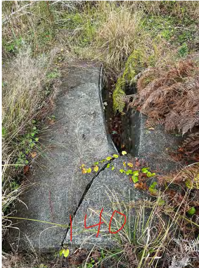
Pond 140 Outfall – Repair cracked structure. Clear Vegetation
